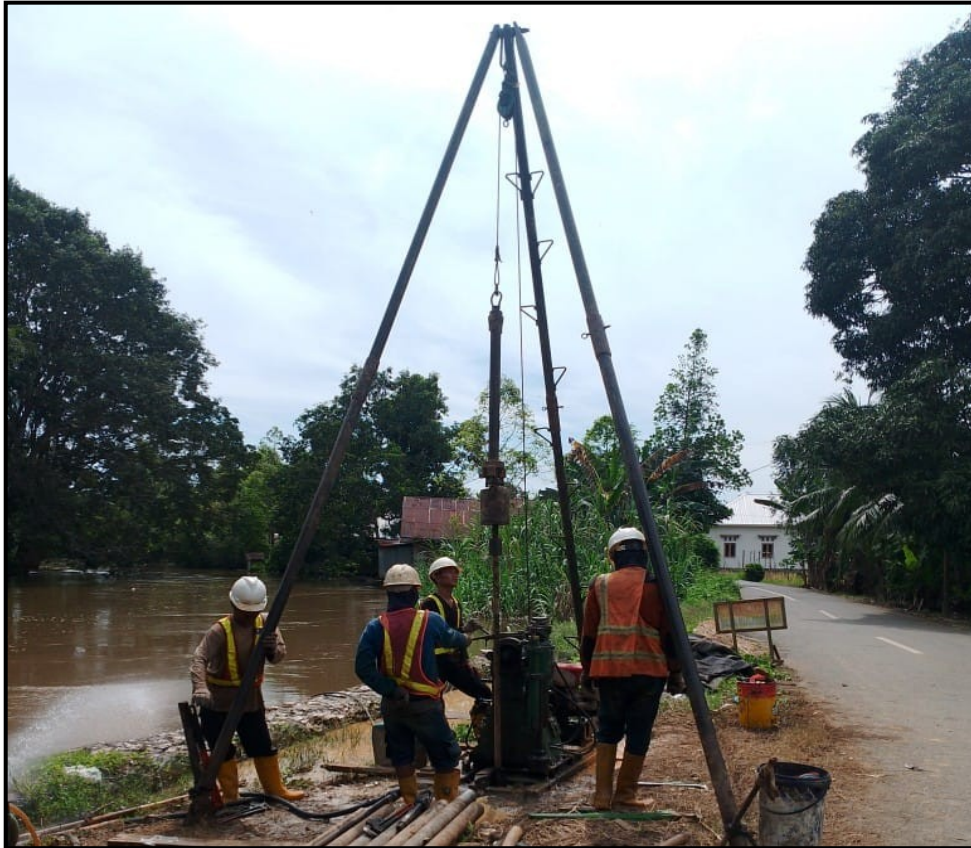
Gambar 1. Dokumentasi Standard Penetration Test
